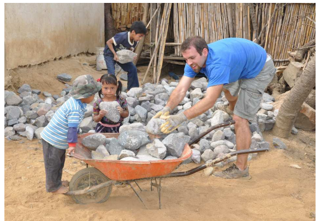
Hauling rocks for the foundations of the house
