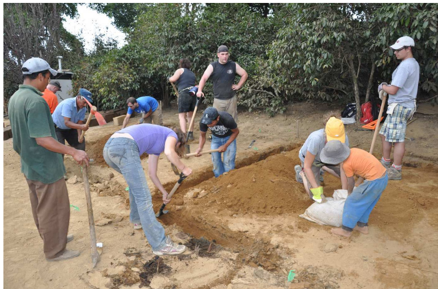
Digging trenches for the house foundations
