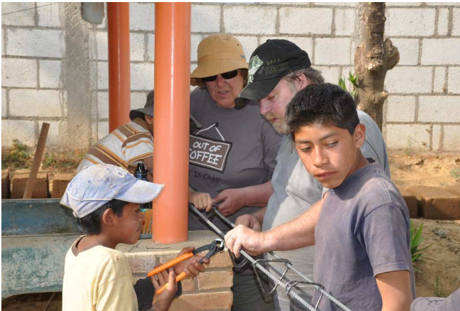
Wiring the rebar
